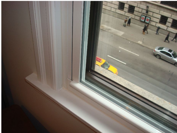
STYLE #14 (DOUBLE HUNG WINDOW) BAKED WHITE ENAMEL PAINTED WINDOW IN FRONT OF A DARK BRONZE ANODIZED WINDOW
