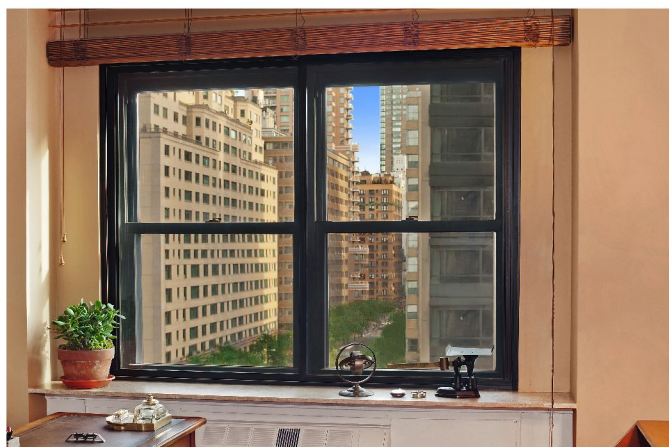
STYLE #11 (2-PANEL SLIDER) DARK BRONZE ANODIZED ALUMINUM WINDOW IN FRONT OF (2) DOUBLE HUNG WINDOWS IN ONE OPENING
