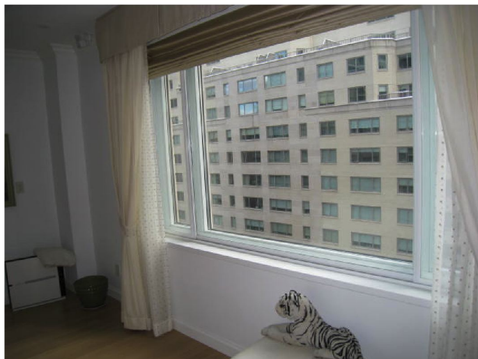
STYLE #15 (3-PANEL SLIDER) BAKED WHITE ENAMEL PAINTED WINDOW IN FRONT OF (3) WINDOWS IN ONE OPENING
