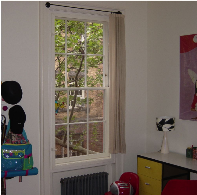
STYLE #12 (HINGED UNIT) BAKED WHITE ENAMEL PAINTED HINGED UNIT WINDOW IN FRONT OF A WHITE DOUBLE HUNG WINDOW. A GOOD CHOICE WHEN SILL DEPTH IS LIMITED.
