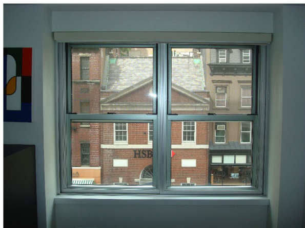
STYLE #11 (2-PANEL SLIDER) CLEAR ANODIZED ALUMINUM WINDOW IN FRONT OF (2) DOUBLE HUNG WINDOWS IN ONE OPENING
